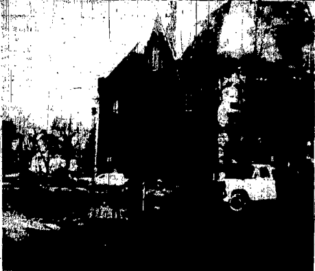
FIRST WORK on the new county jail and sheriff's residence got underway before the storm. The site is northwest of the turreted courthouse.
